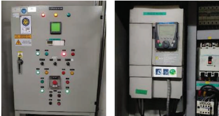
UID – Installation of VSD in cooling system.
