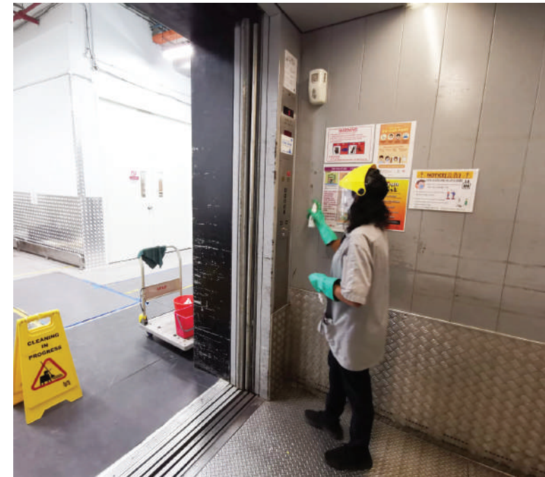
USG – Applying SDST antimicrobial coatings at common touch areas.
