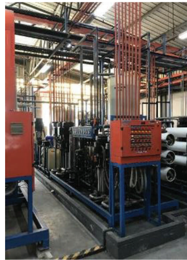
UTL3 – Recycled reject RO water by increasing quality and supply water to feed RO system (top and bottom images).
